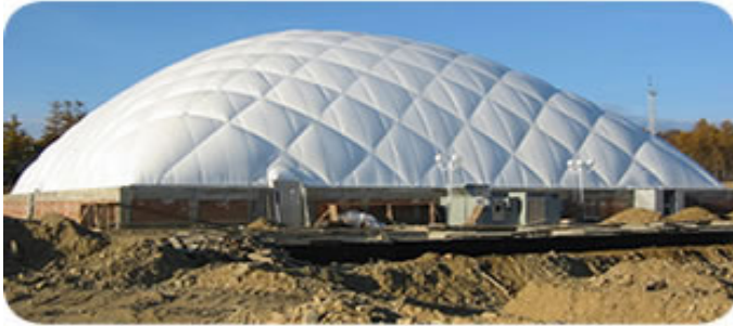
Construction Site Enclosure
