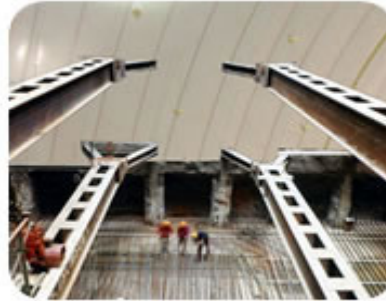
Interior Work Site
